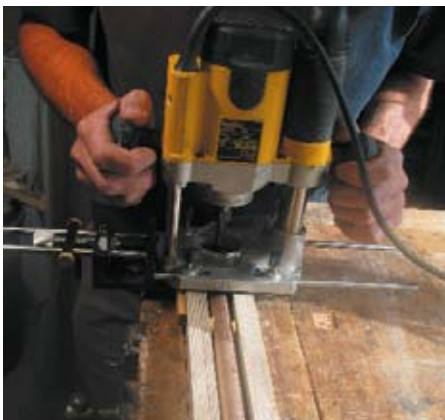
Set-up for routing the groove
