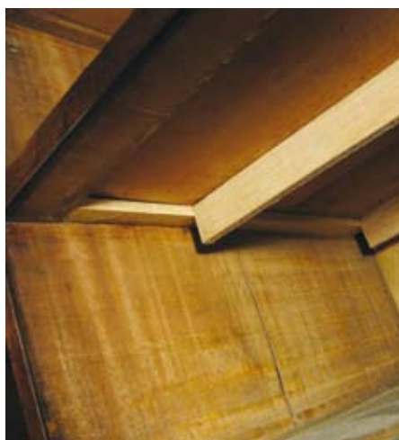
9 Kicker being glued in place; sprung lathes hold it in place
