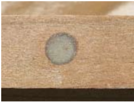
The magnet fixed in the cabinet side with epoxy, then cleaned up
